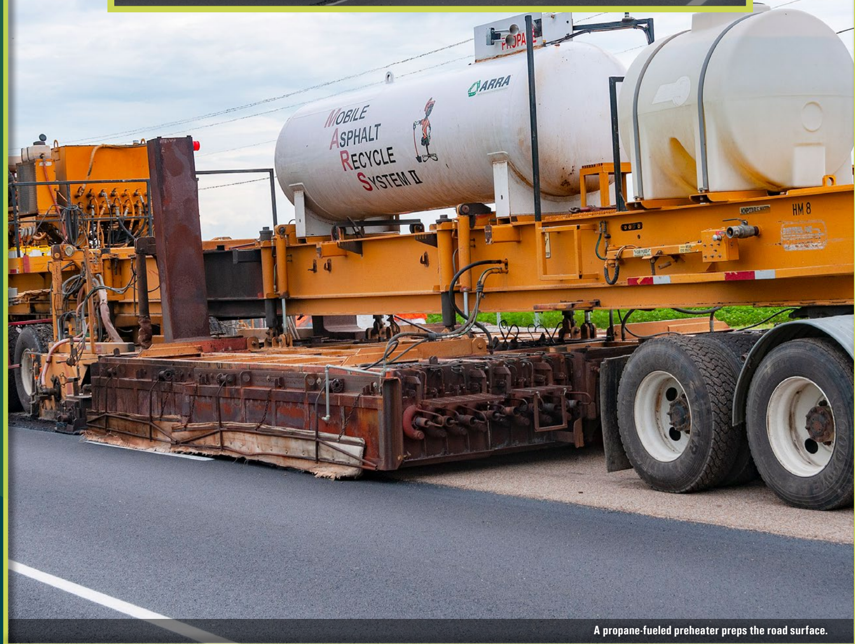
The equipment "train" only utilizes one travel lane.
